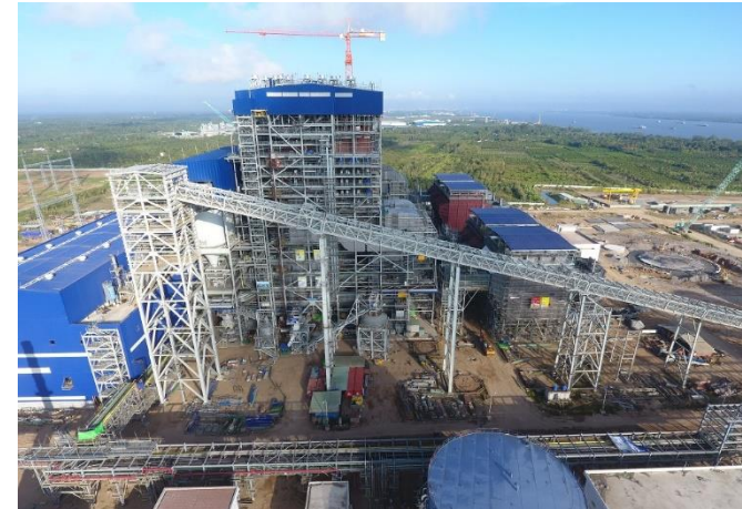
Installation the CHS
