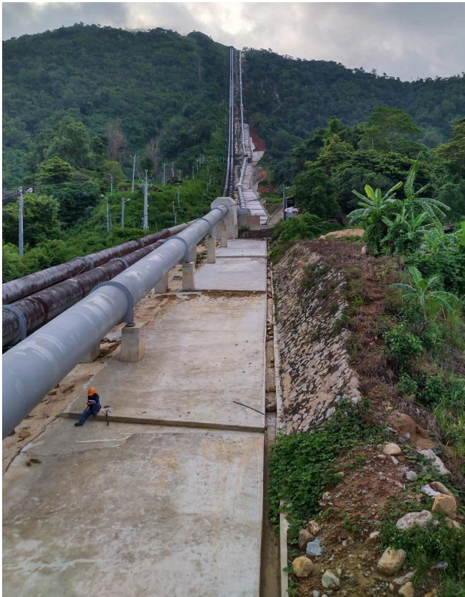
Penstock for Extension Da Nhim hydropower plant project
