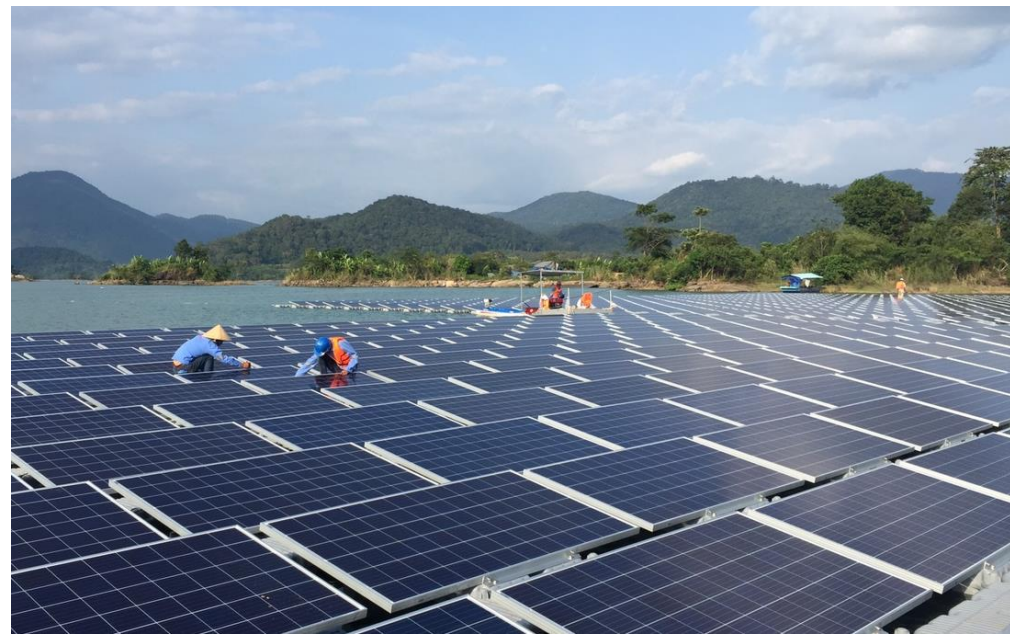
Buoy installation for Da Mi floating solar power plant project
