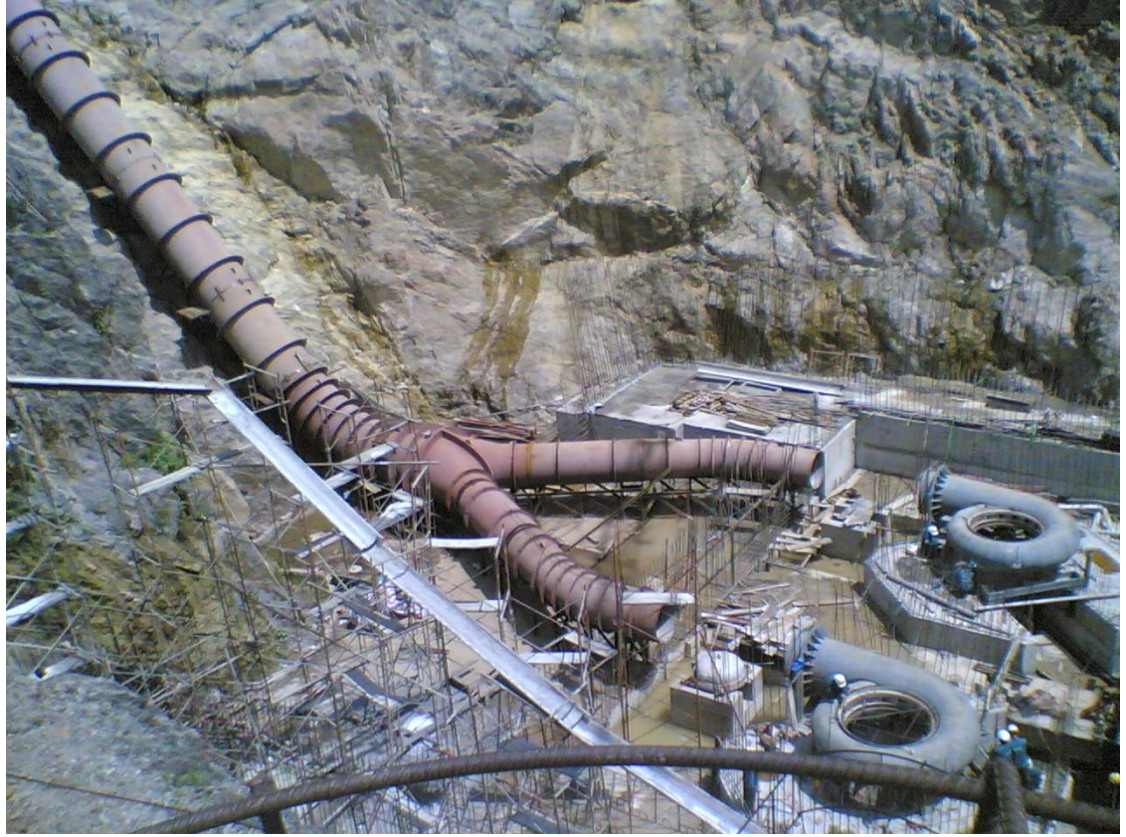
Penstock for Extension Da Nhim hydropower plant project
