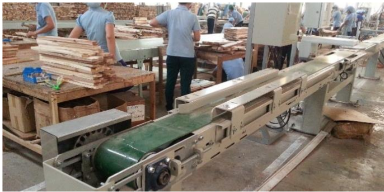
Wood board moisture classification system controled by PLC S7-1200
