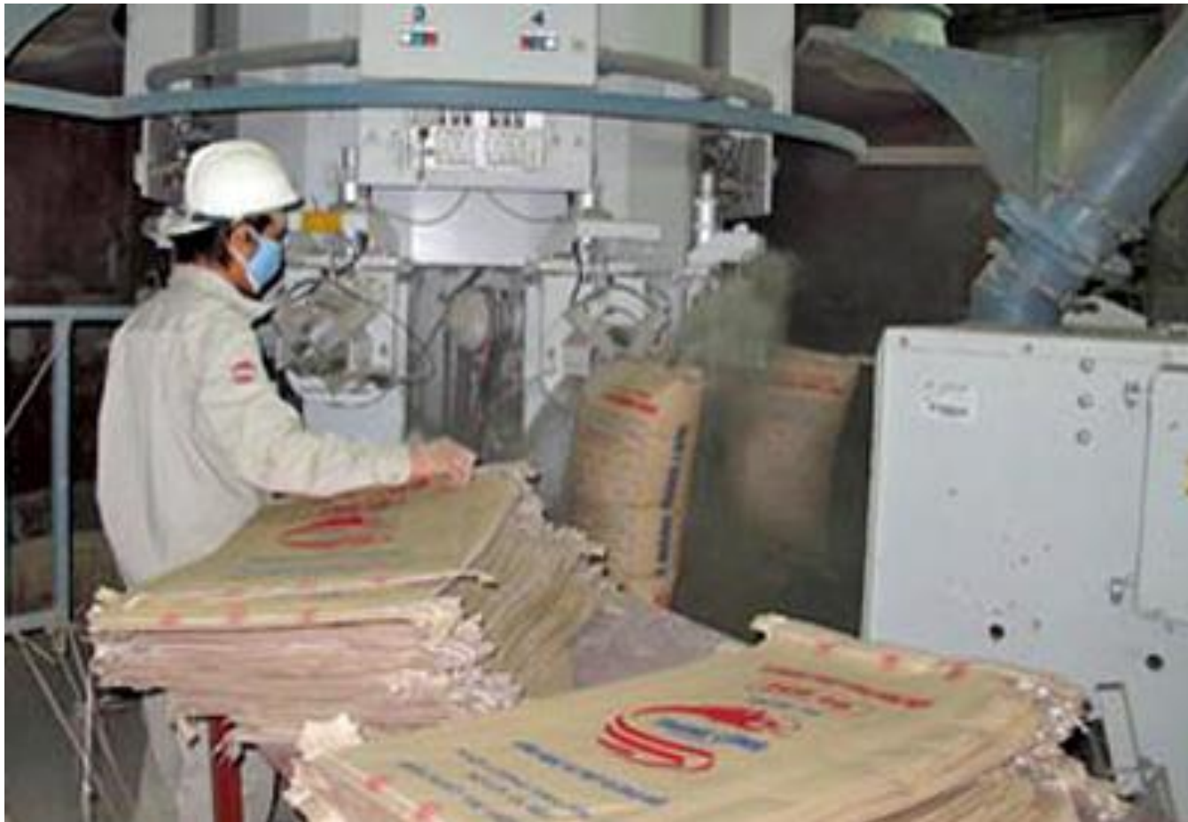
Packaging system for cement plant
