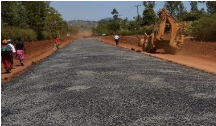
Construction of 300 km road project in Meru County, Kenya
