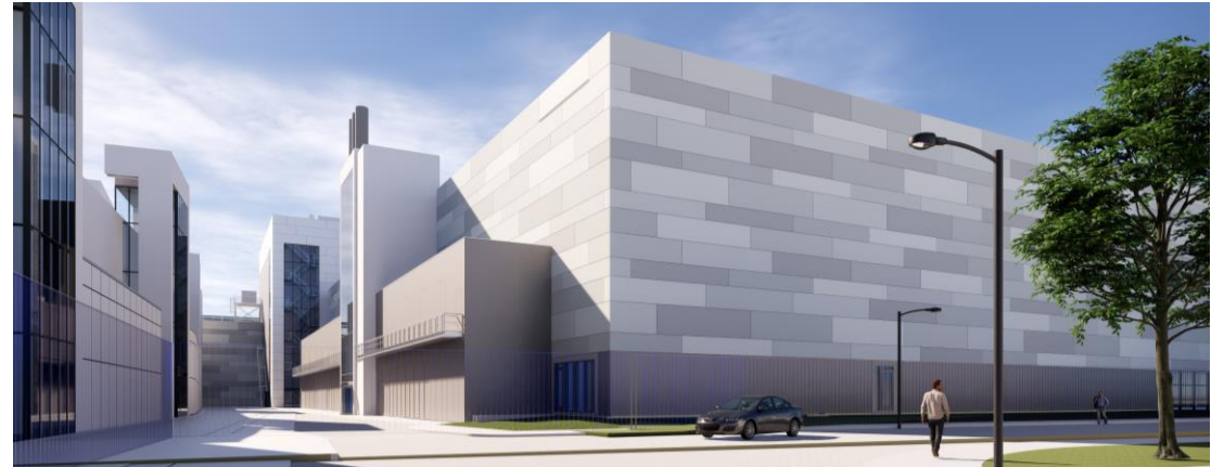
High-NA cleanroom under construction on ASML's campus in Veldhoven
